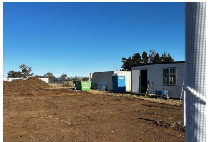
A security fence with visual wrapping has been installed.
